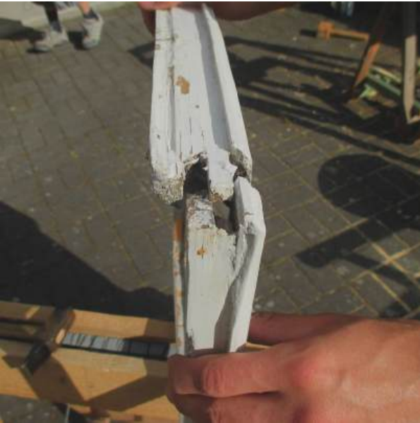
Abb. 6: Lockere Eckverbindung
